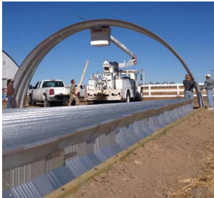
Hay Barn: The Giant Erector Set in Progress.
